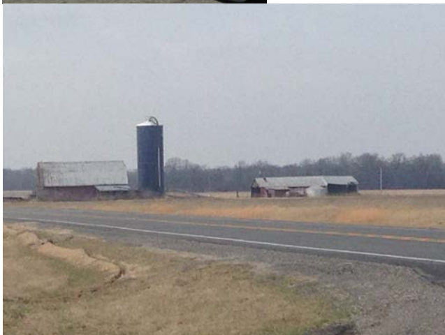
Signs of Decay: Farm structures along Highway 50 that are in disrepair.
