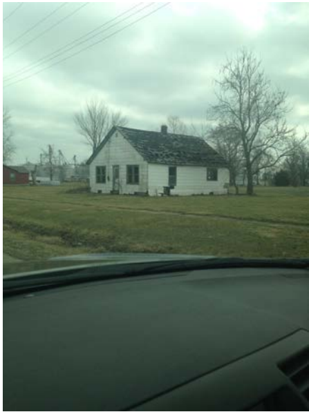
Signs of Decay: Home that appears to be abandoned with overgrowth
